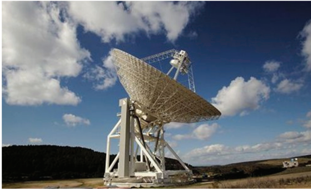
Fig. 2. The Sardinia Radio Telescope (SRT) as receiver of the BIRALET system.
