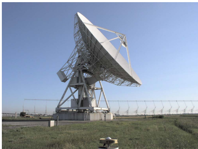
Fig. 1. 32-m AZ-EL VLBI radio telescope at Medicina; the VLBI telescope in Noto has the same design, structure, and dimensions
