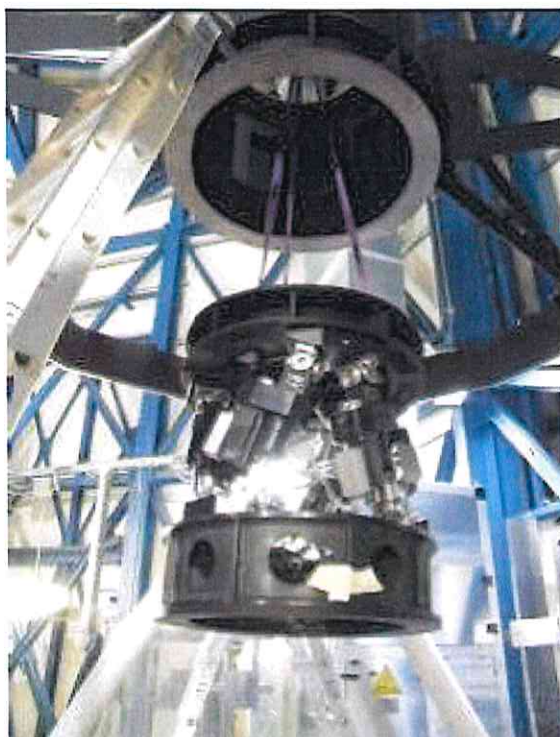
Fig. 6 – A phase of the installation of the hexapod in the telescope.
