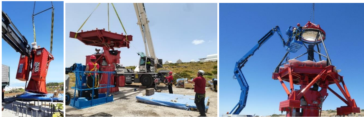
Figure 6. Mounting of the first ASTRI Mini-Array telescope at the Teide observatory. Left: The mounting of the base of the telescope on the foundation. Centre: The mounting of the M1 dish on the azimuth fork. Right: The mounting of M2 support structure (courtesy of EIE Group).
