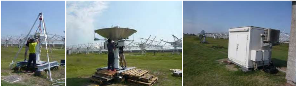
Fig. 2: Installation of transportable VLBI station at Medicina. The transportable 2.4 m antenna consists of separate assemblies for the dish and Az/EI drive system. Three persons are sufficient to assemble the system in two days of work (Left and Center). A small air-conditioned box, located 30 m from the antenna, contains antenna control system(right).
