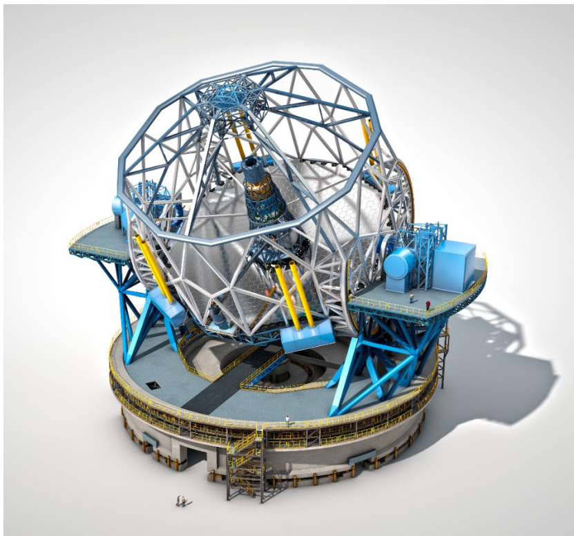
Figure 1. The Extremely Large Telescope (credit ESO) will be the largest optical telescope in the world, with a primary mirror diameter of 39.5 m. Instruments, will be fed from ports on one of the Nasmyth platforms (here shown left and right). The optical spectrograph of HIRES will be located on one of these platforms, with the NIR spectrograph located below in the Coudé room.
