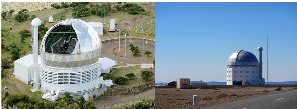
Figure 1. Towers are employed to house the Center of Curvature Calibration Sensors, to align the mirrors of the Hobby-Eberly Telescope (left) and of the Southern African Large Telescope (right).
