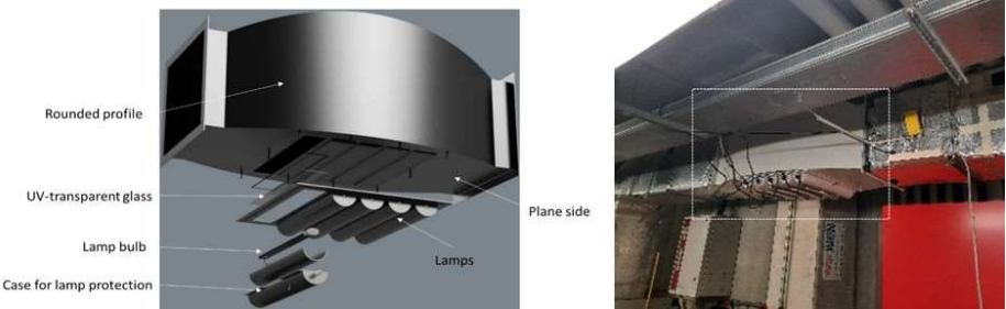
Fig. 1. Left: exploded 3D image of the system designed for installation in the existing ATU duct at CSMT Headquarters and adapted from (Lombini et al., 2022). Right: Prototype installed at CSMT Headquarters.
