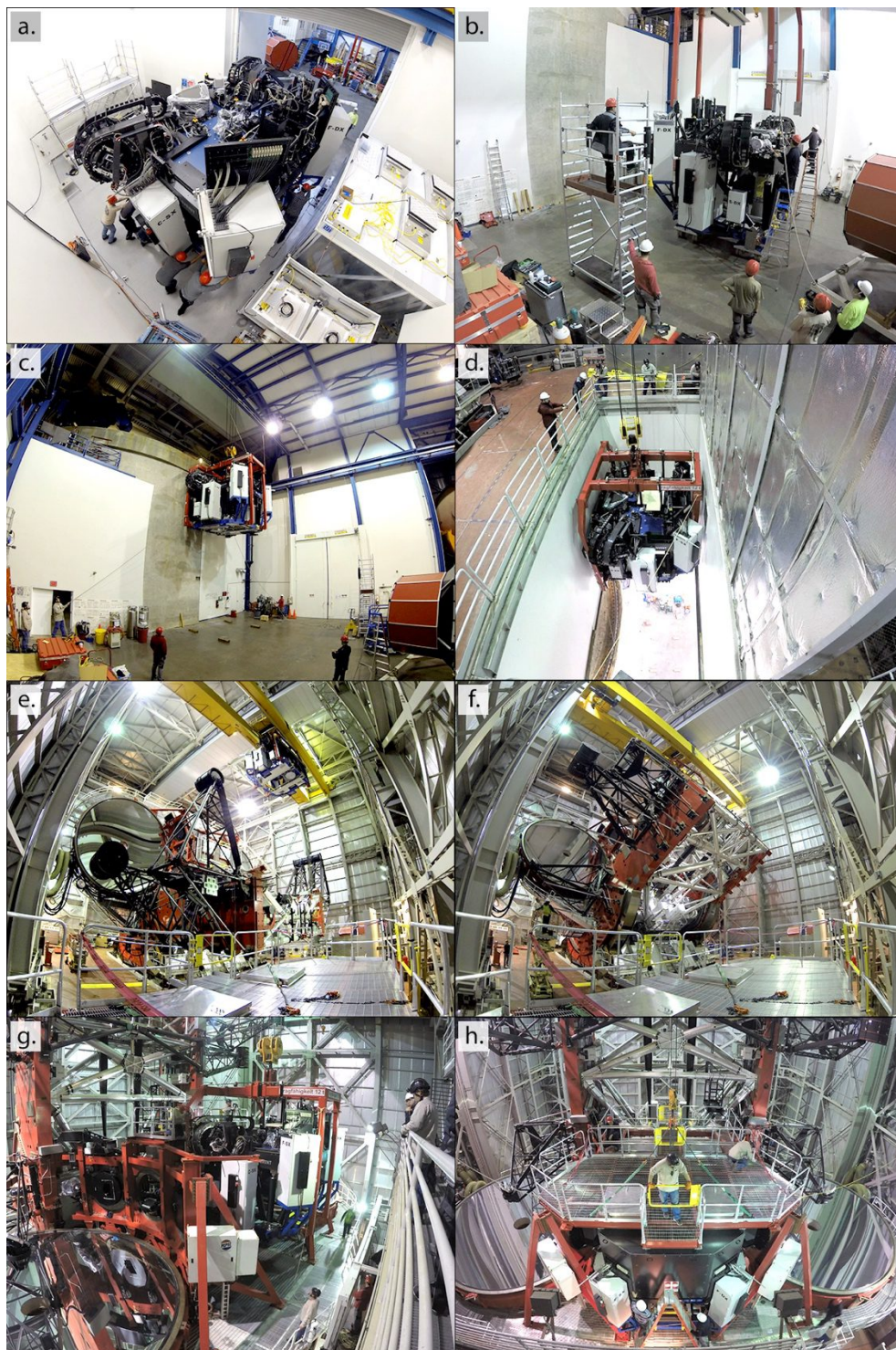
Figure 1. Final installation of LINC-NIRVANA on the LBT. The team pushes the instrument out of the mountain lab (panel a) and into the high bay, where the bridge crane assists in installing the lifting traverse (panel b). Flying the instrument from the high bay into the enclosure is an interesting challenge, since the clearance between instrument and building is only about 11mm (panels c and d). A well-choreographed “dance” with the telescope (panels e and f) allows LINC-NIRVANA to travel to the rear of the enclosure to its final mounting location (panel g). A similar dance brings the dust cover and “roof garden” into place (panel h). The entire operation took two full days.
