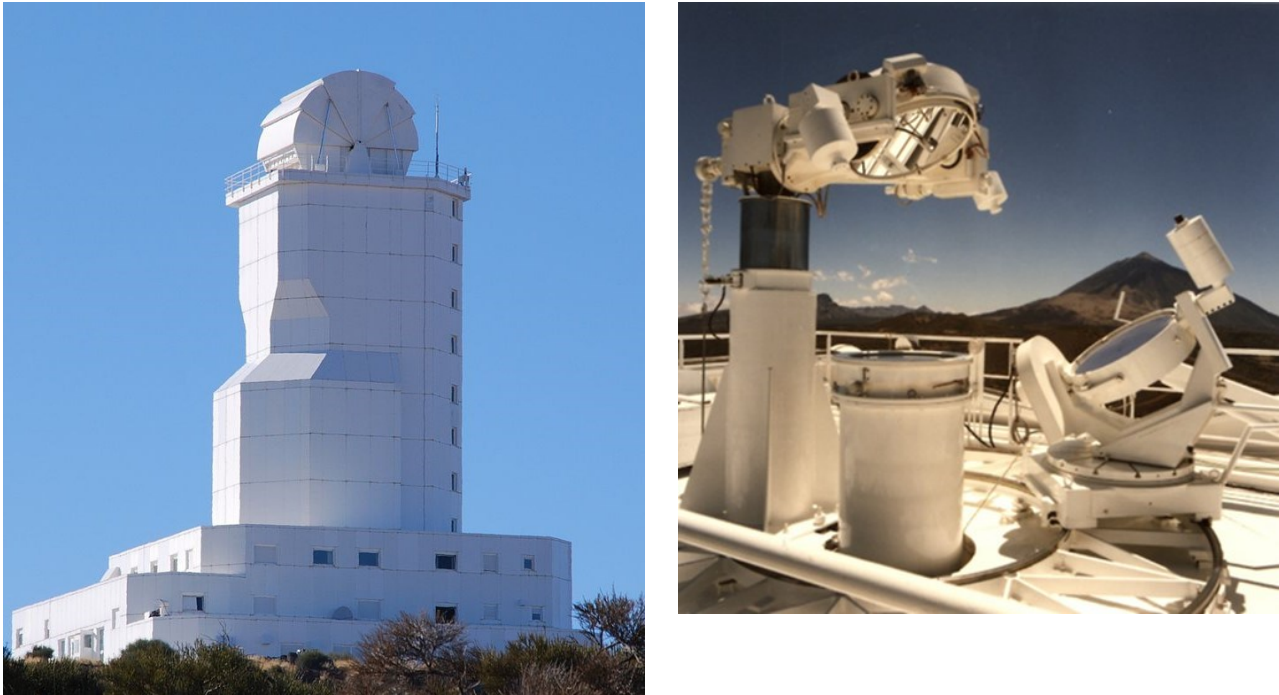
Figure 1: VTT building (left) and the coelostat (right).
