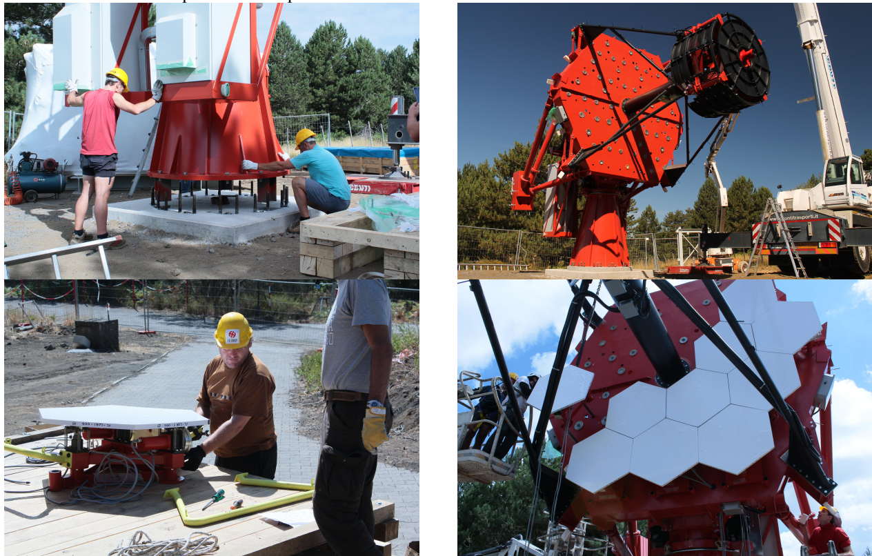
Figure 4: Highlights of the telescope opto-mechanical on-site installation. (top-left) Positioning and alignment of the mount assembly on the foundation (top-right) Completion of the telescope structure (bottom-left) Primary mirror segments and active optical support integration (bottom-right) Primary mirror installation.
