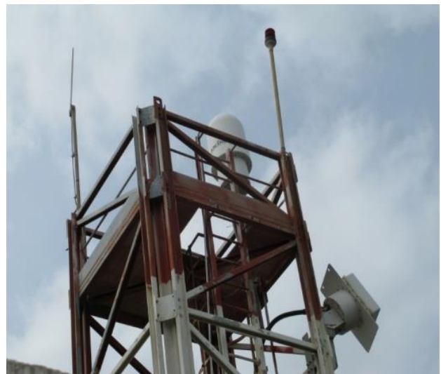
Figure 2. The “Flight Termination System” (FTS) transmitter
