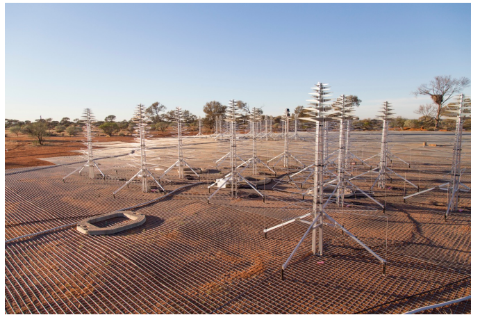
Fig. 2. The AAVS1.5 array on the Murchison Radio-astronomy Observatory, May 2019, showing a close-up view of one of the 16 SKALA4.1 antenna clusters. Credits: ICRAR/Curtin.
