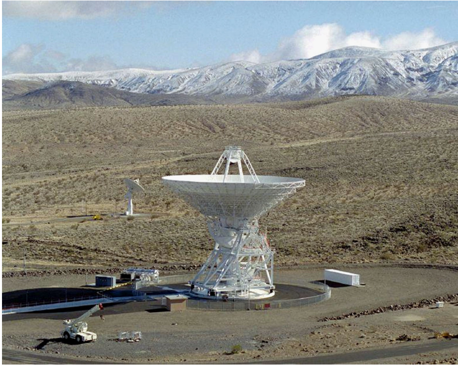
Fig. 3 NASA/JPL Deep Space station 25 (DSS25), a 34-m beam waveguide antenna, shown here in the stowed position. It was specifically instrumented for Cassini radio science with high-stability electronics, Ka-band up-and downlinks, and advanced media calibration systems to correct for tropospheric scintillation (credit; NASA-DSN)
