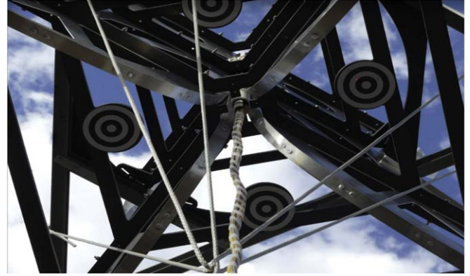
Figure 13. A view of the underside of a Vivaldi feed, showing the targets for the leveling jig. This jig ensures that the feed is positioned correctly using a laser plumb bob. The cable wrapping coming from the feed center extends to the bottom of the image.
